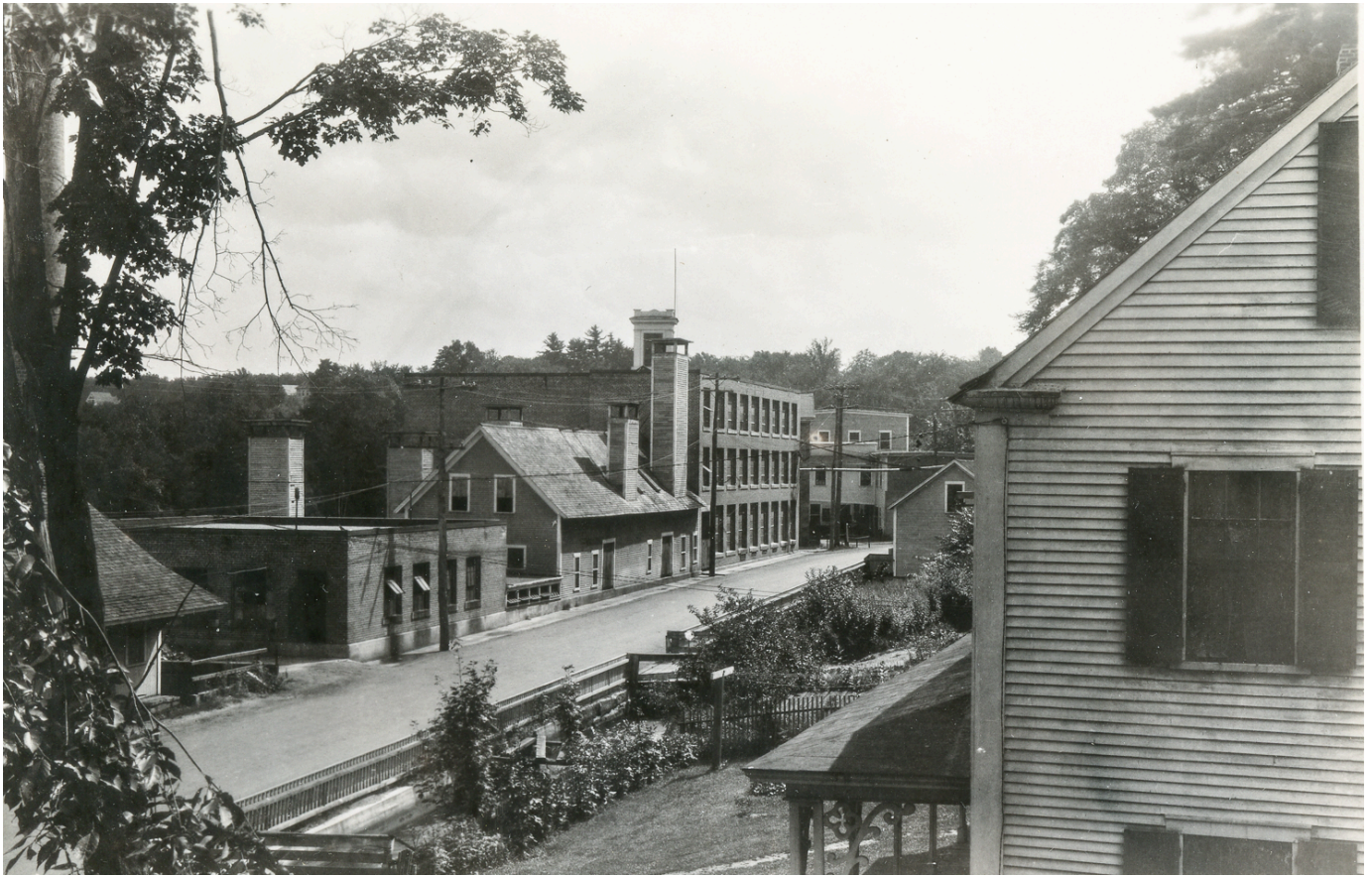
Looking south on Commercial St. Harris - Emery Woolen Mill c. 1940
