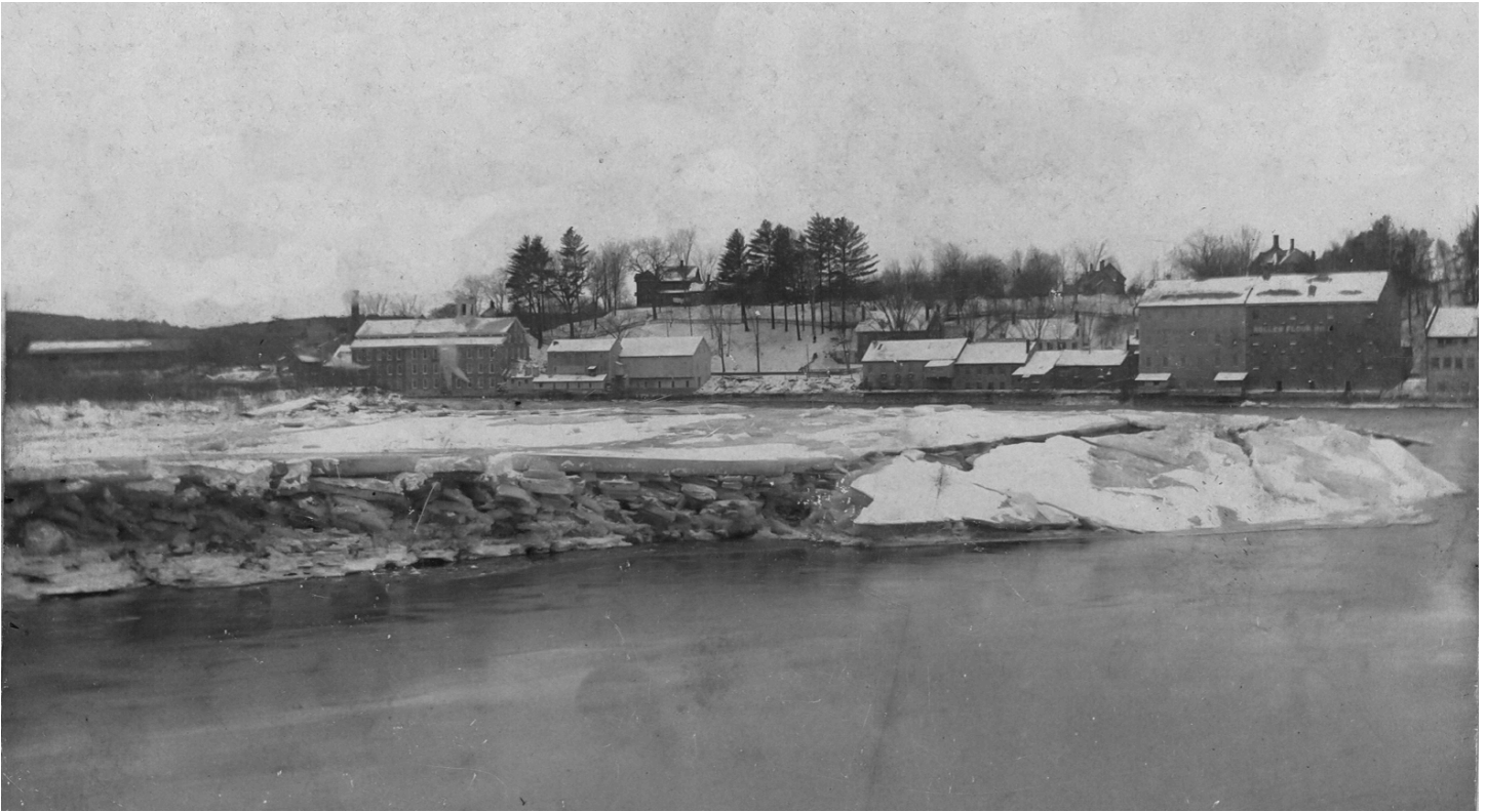
View from Dustin Island – Stratton & Co. on the right, Harris-Emery Woolen Mill on the left c. 1890
